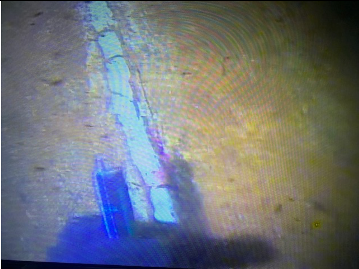
Fig. 2 Leak test west slope midway
