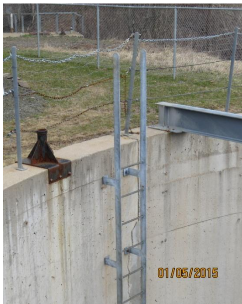
Ladder system to be modified to meet NS OH&S
