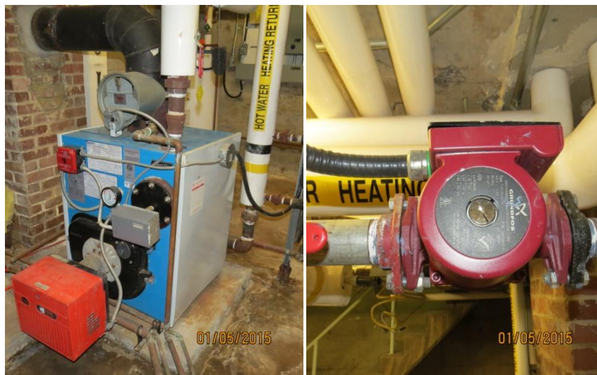
Slant-Fin boiler and Riello burner
