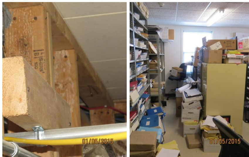
At Council Chambers, hall side, Not fire sealed
