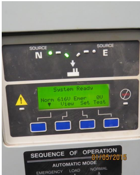
Transfer switch- systems normal and ready
