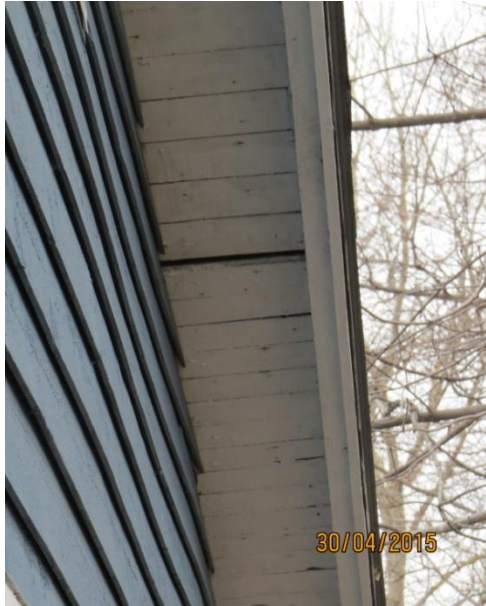
Minor repairs to wood soffit required
