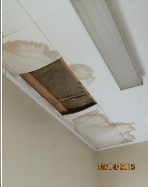
storage room roof leak
