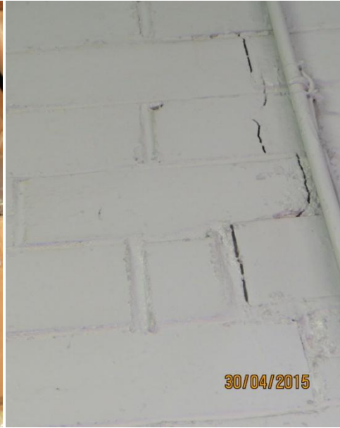
typical structural crack
