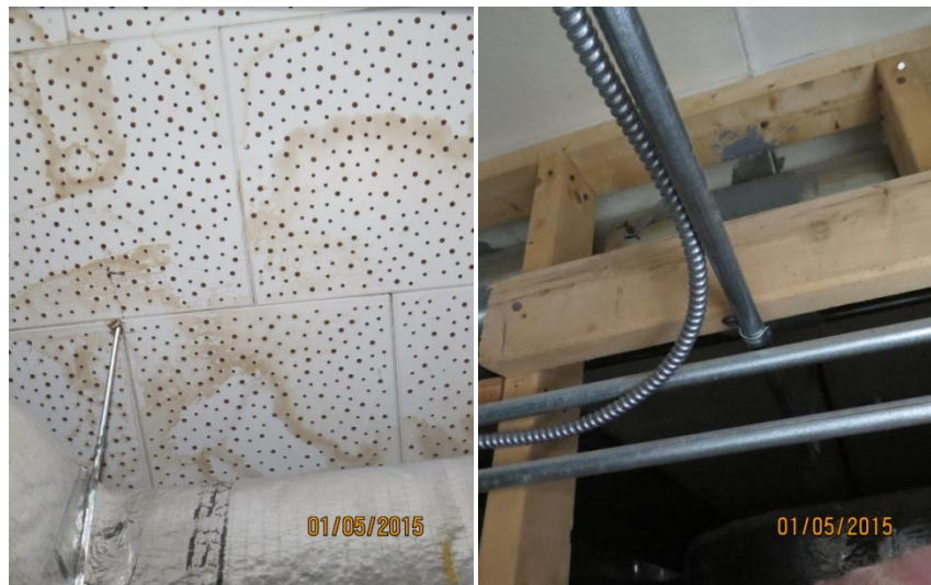
Area above upper floor ceiling, water leaks (roof leaks) on upper ceiling tile, upper ceiling tile may contain asbestos, means of egress halls not fire separated or sealed
