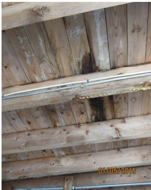
Leaking roof
