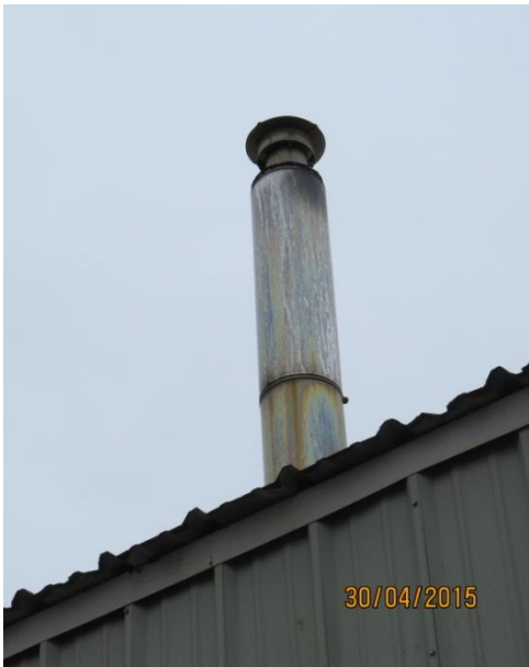
Heating system exhaust
