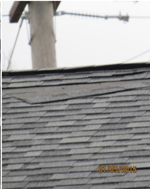
Front elevation- lose shingles
