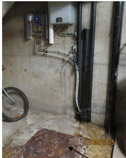
Decayed cover on sump pit
