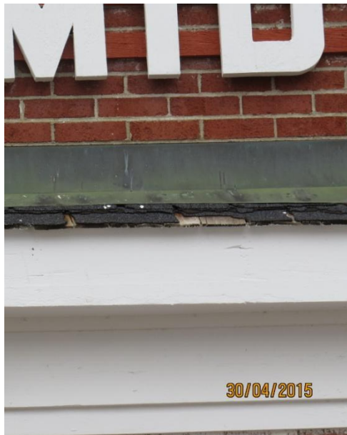
Flashing and shingle failure above vehicle door
