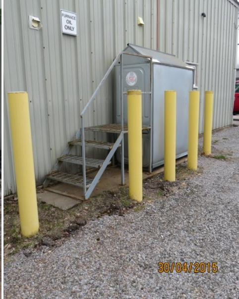
Double wall furnace fuel tank-heating
