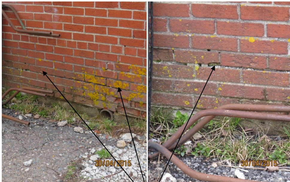
Mortar and brick decay- non structural
