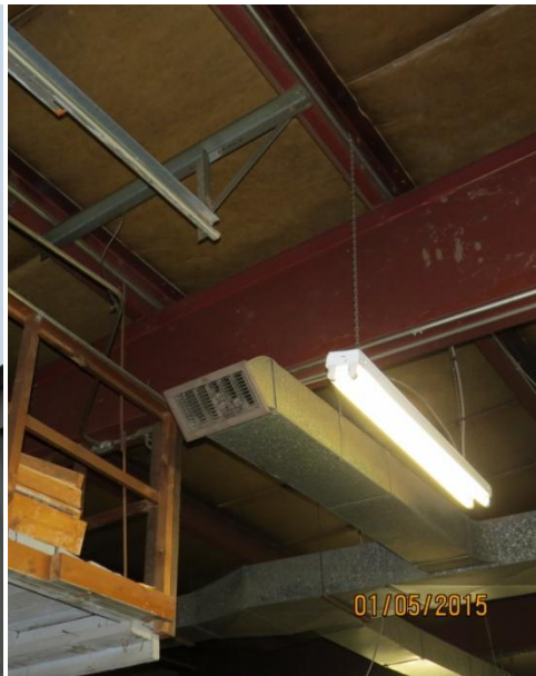
typical forced air heating duct work
