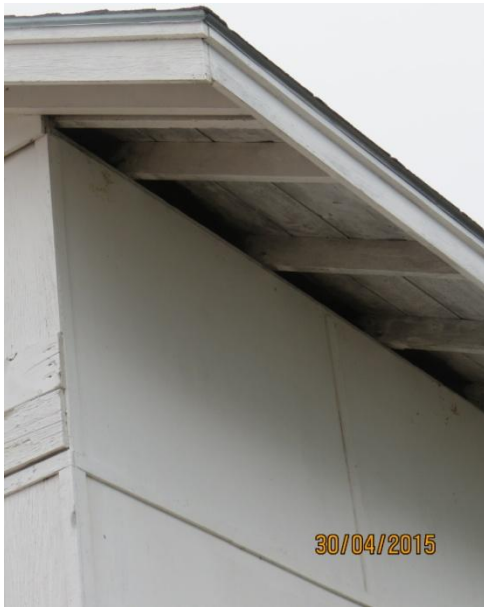
Open soffit ventilation
