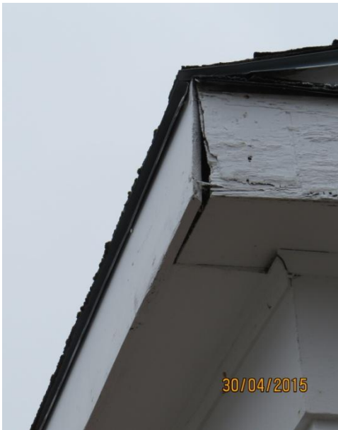
extensive decay to fascia and flashing
