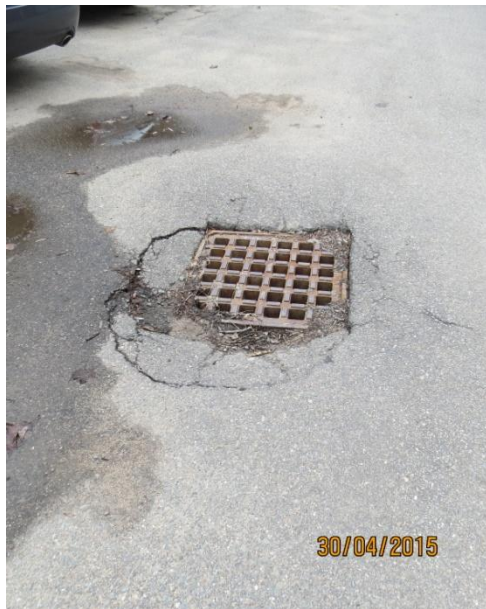
East side catch basin needs repairs
