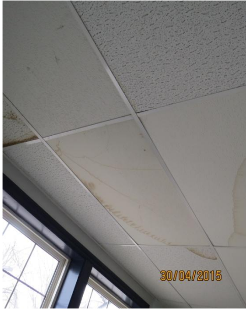
Ceiling tile damage- leak above
