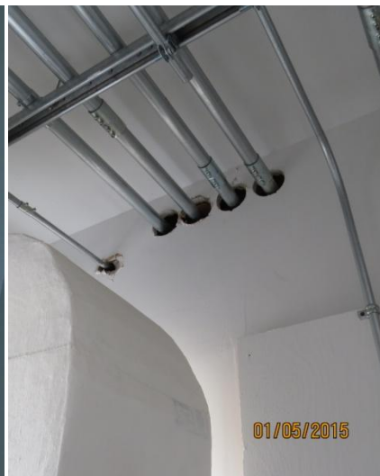
electrical pipes not sealed
