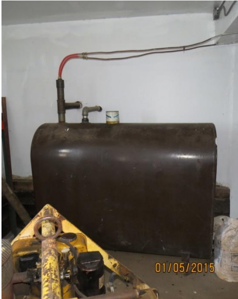
Unit 2 heating fuel- not to Code
