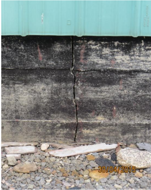
Foundation crack
