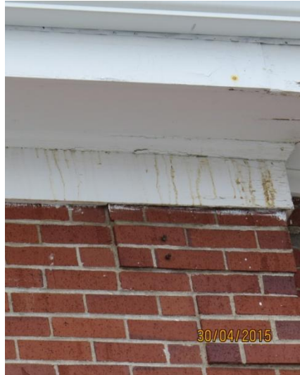
Asphalt leakage behind fascia- roof replacement required- see main building details
