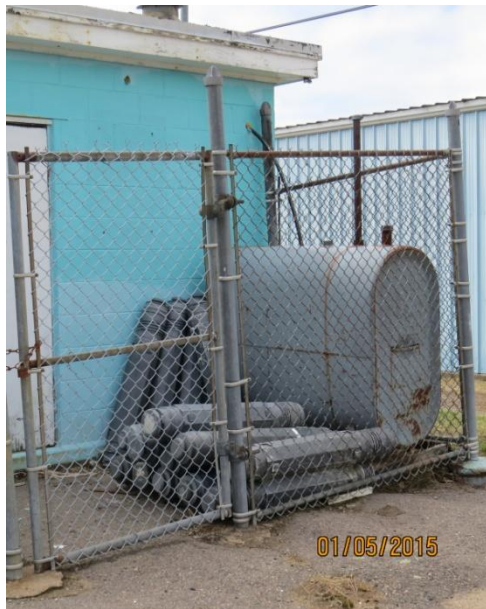
Replace 909 litre single wall tank
