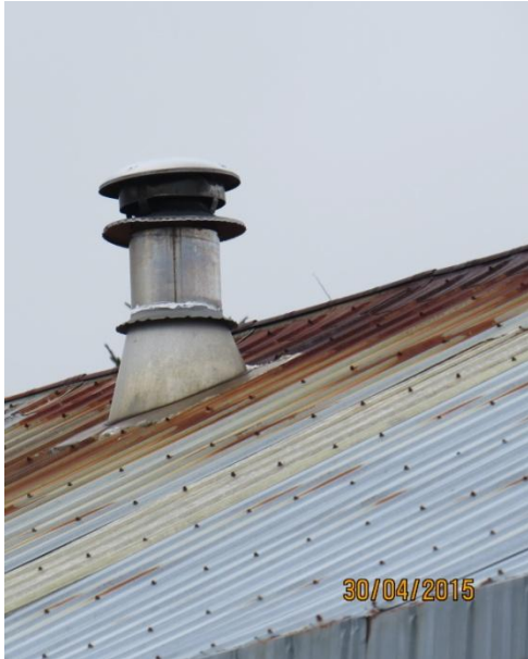
Rusted roofing system
