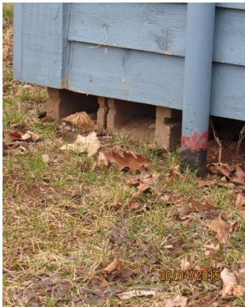
Concrete block footings have shifted
