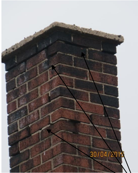
Structural deflection and mortar decay
