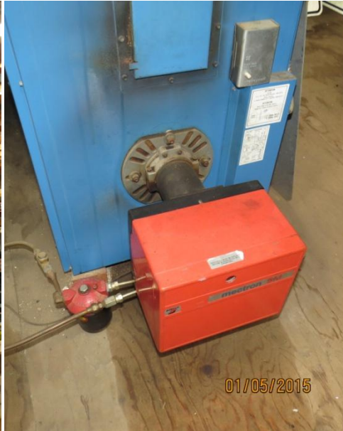
Mectron burner
