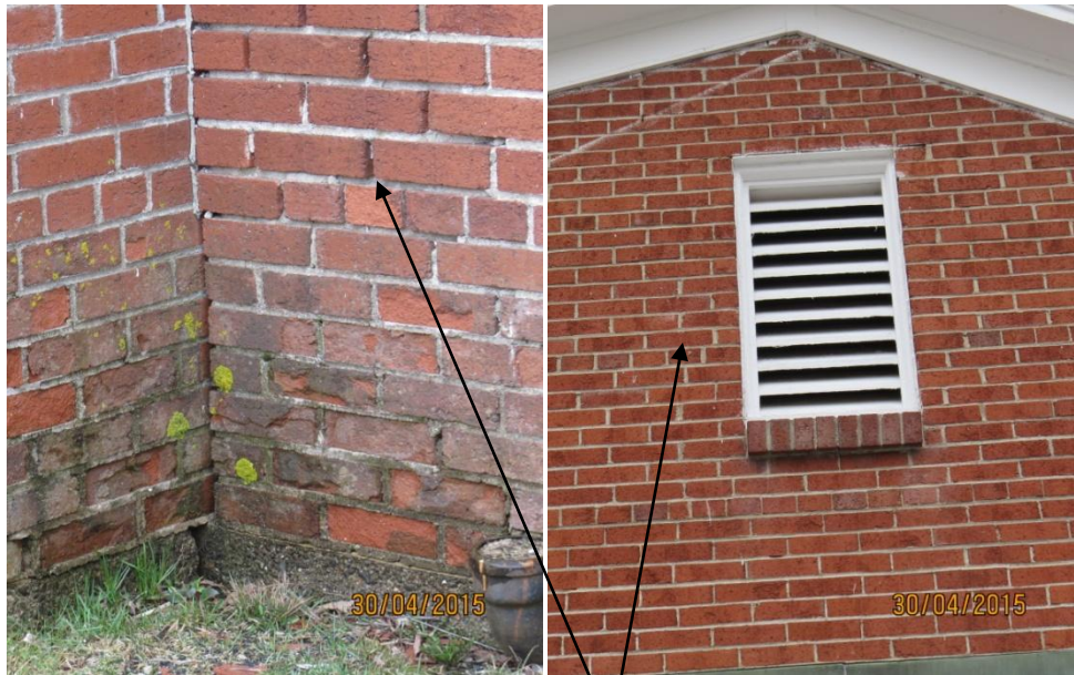
Mortar and brick decay- structural deflection
