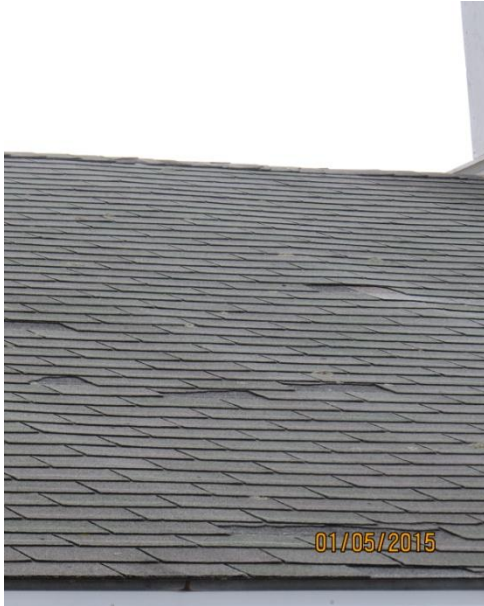
West side roof several shingles missing
