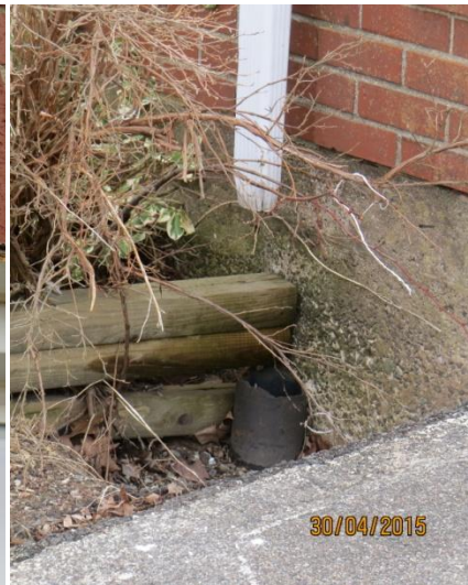
downspout not connected to drain
