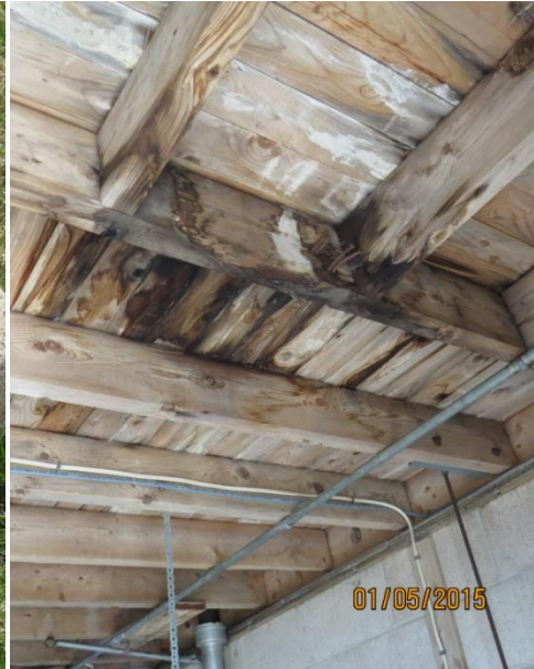
Leaking roof
