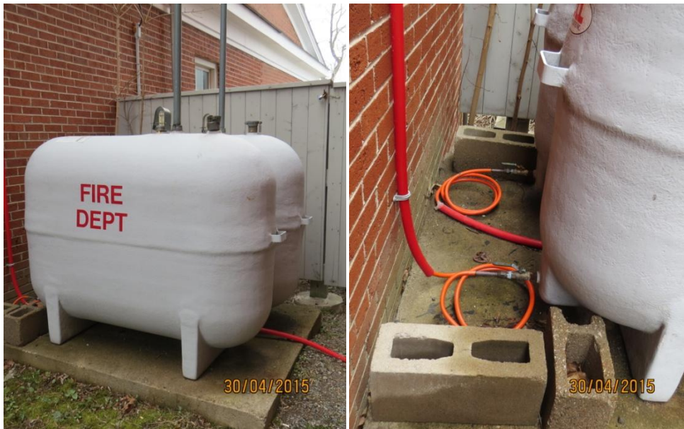
Heating fuel storage tanks
