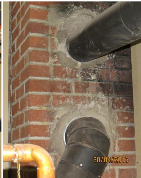
boiler exhaust leaking
