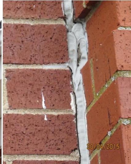
expansion joint requires repair
