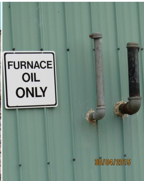
heating system fuel tank fills and vent pipe
