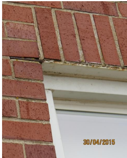
Steel lintel requires repair
