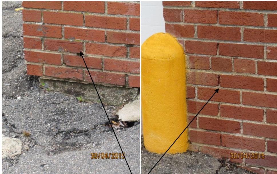
Mortar and brick decay- non structural
