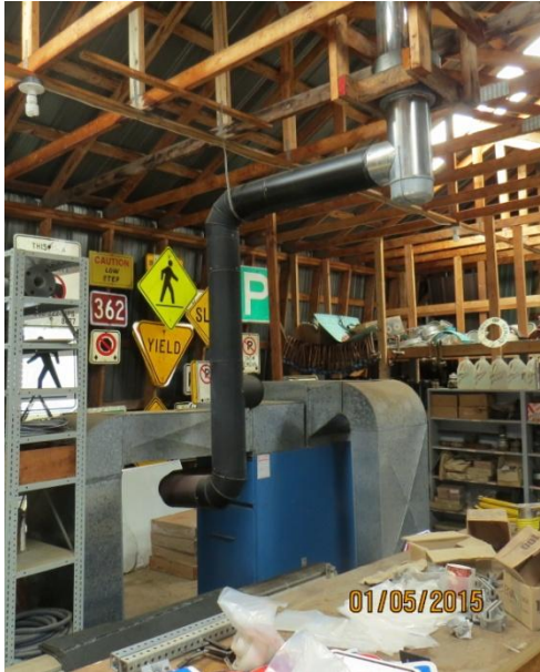
Gemini boiler and ventilation
