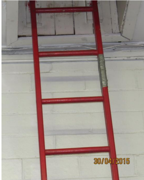
Broken attic access ladder- duct tape on vertical
