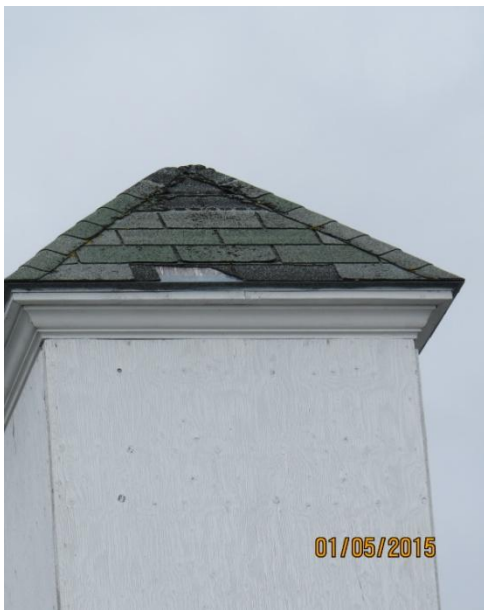
Tower on roof- shingles missing
