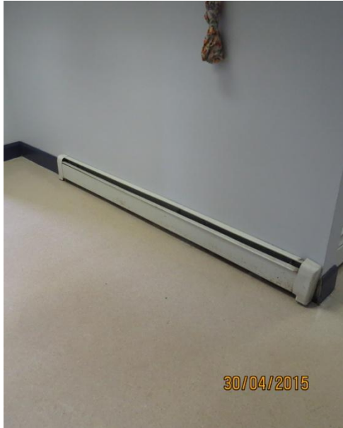
Typical hot water baseboard heater
