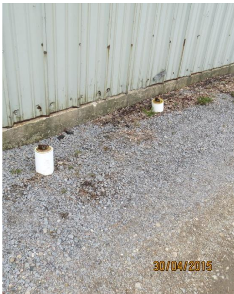
Former refueling center monitoring wells
