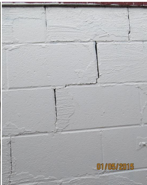
Cracks in east wall
