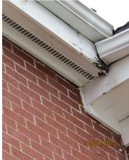
Misc. Wood decay at roof eave
