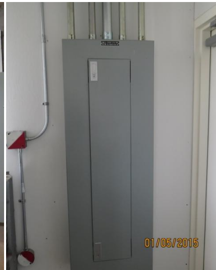
secondary distribution- upper floor
