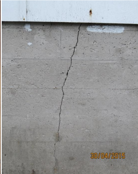
Structural crack in foundation
