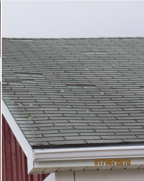
east roof- several shingle missing
