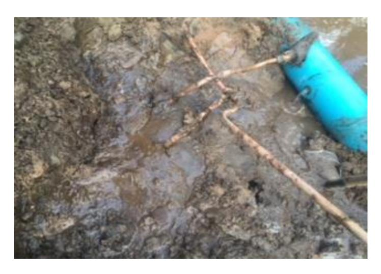
Service attachment failed. The line is in fairly good condition however the service connections are failing. When the excavation was still open a second service connection failed.
