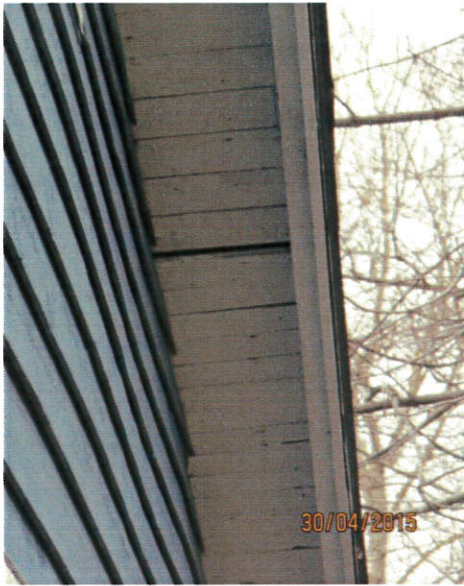
Minor repairs to wood soffit required
