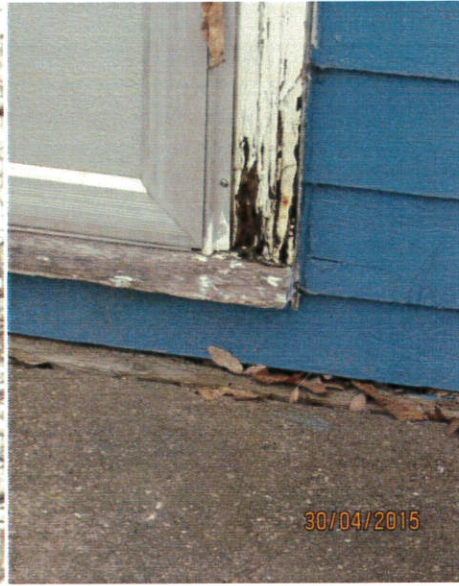
replace wood door and wood frame
