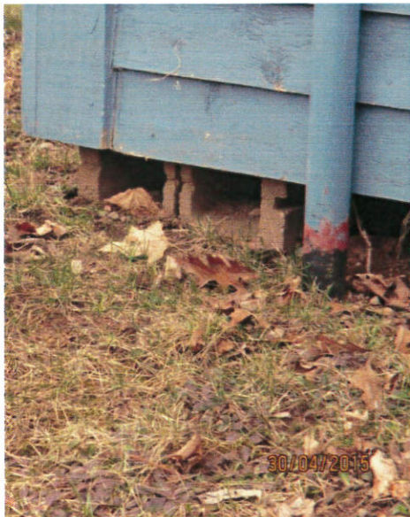
Concrete block footings have shifted
